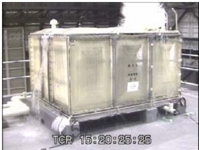
(b-3) Splashing water (Roof)
