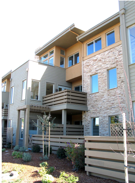
Figure 1. Typical building exterior
