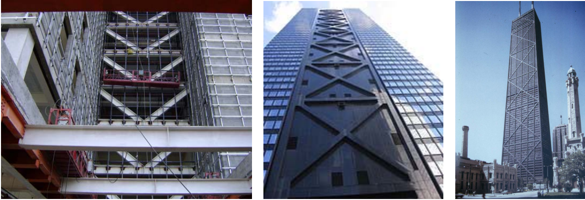
Figure 1. (a) Cross bracing; (b) Mitsui Building, Tokyo; (c) John Hancock Center, Chicago.
