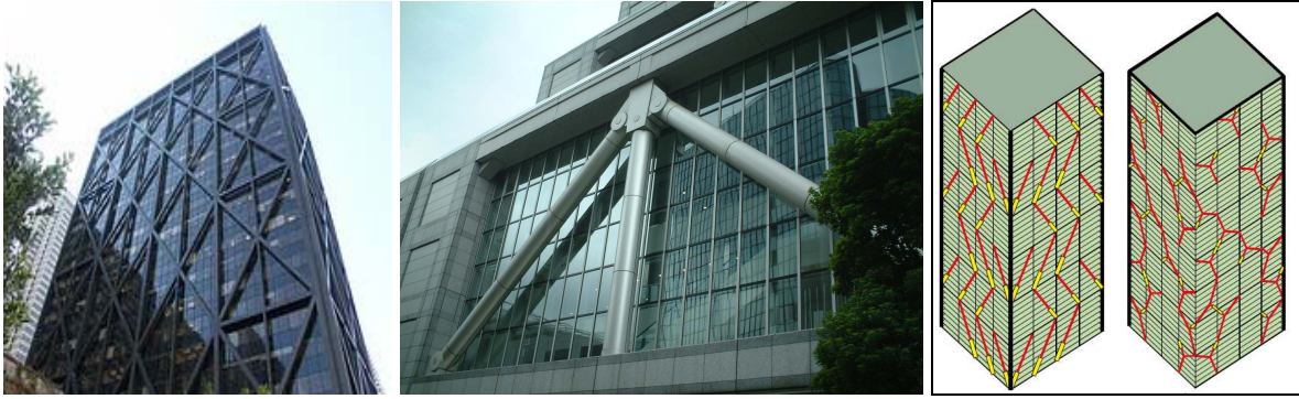
Figure 2. (a) Alcoa Building, San Francisco; (b) United Nation University, Tokyo; (c) Samples of alternative bracing layouts proposed in (Elsesser 2006).
