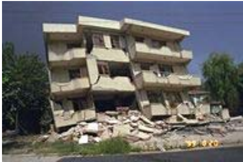
Figure 5. Soft story collapse (Sezen 2000)
