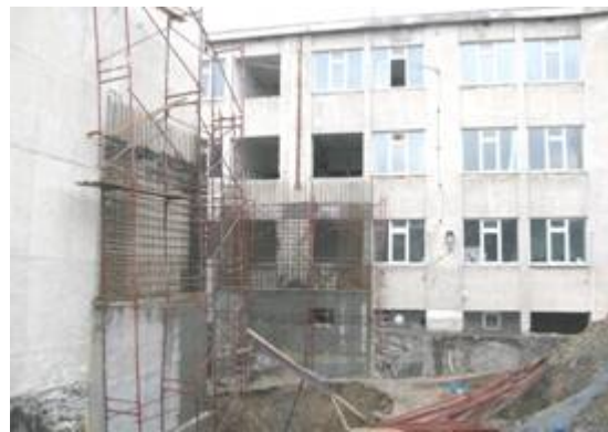
Figure 11. Construction of exterior concrete walls for school retrofit
