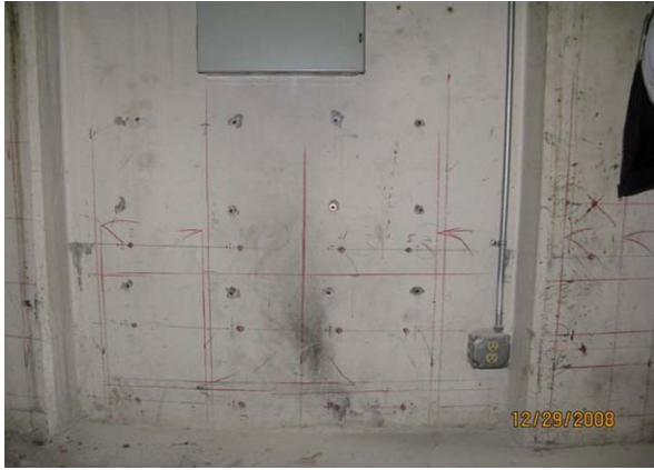
Figure 17. Lap splice retrofit.
