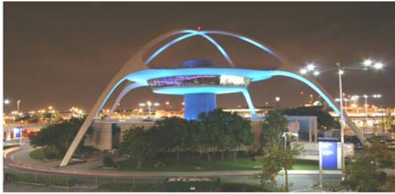
Figure 1. Photograph of the building.
