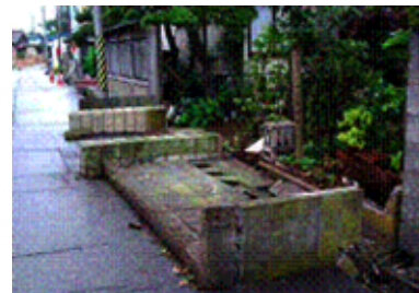
(5) Concrete block wall
