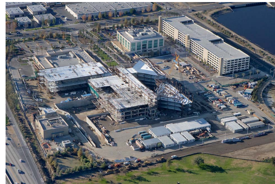
During hospital building construction
