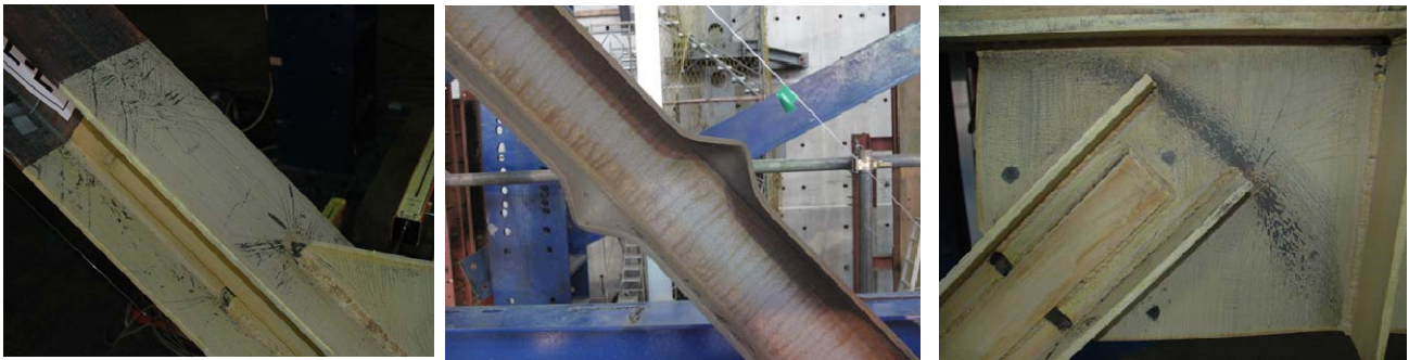
Yielding at Brace Net-Section (-2.43%)
